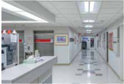
After: Cree TrueWhite® LED Lighting
